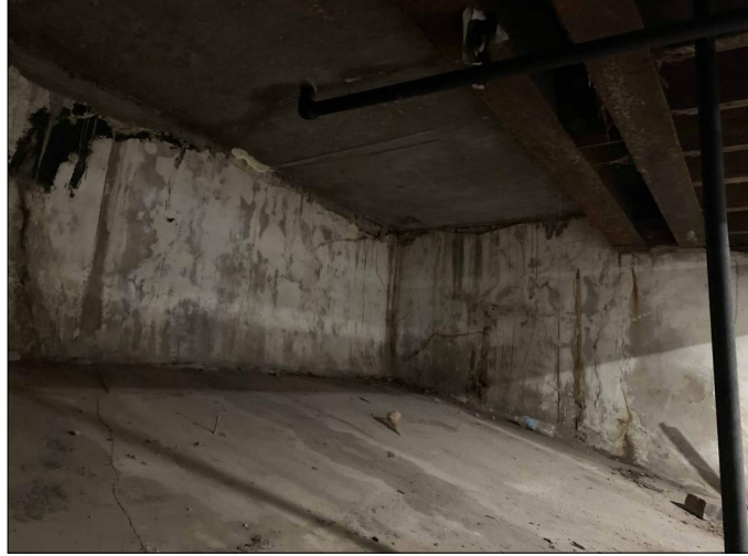
PHOTO 6. BOTTOM OF NORTH VAULT SLAB
