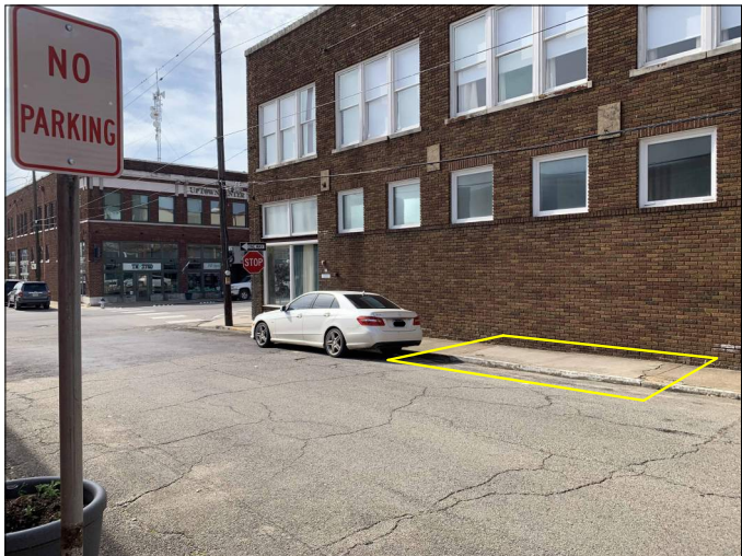
PHOTO 1. SOUTH VAULT FROM OUTSIDE & ABOVE
