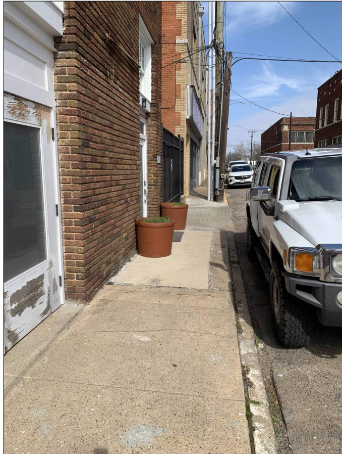
PHOTO 4. NORTH VAULT FROM OUTSIDE & ABOVE
