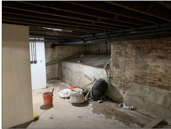
PHOTO 5. NORTH VAULT FROM INSIDE BASEMENT
