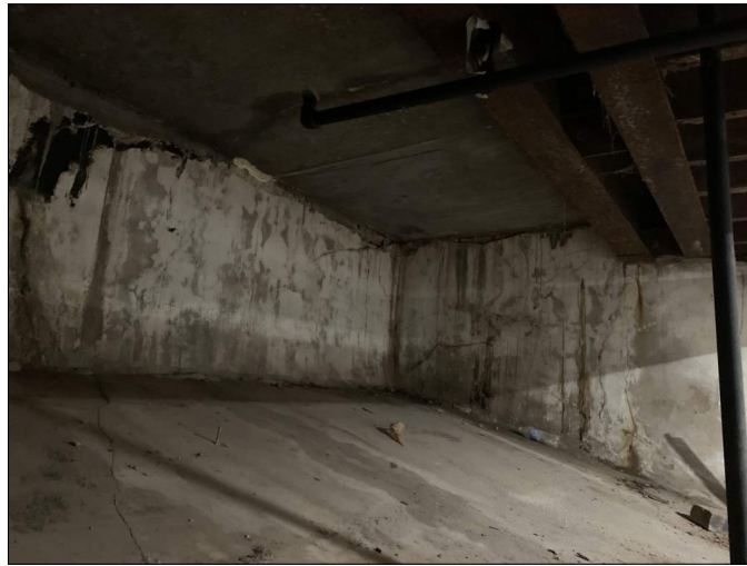
PHOTO 6. BOTTOM OF NORTH VAULT SLAB
